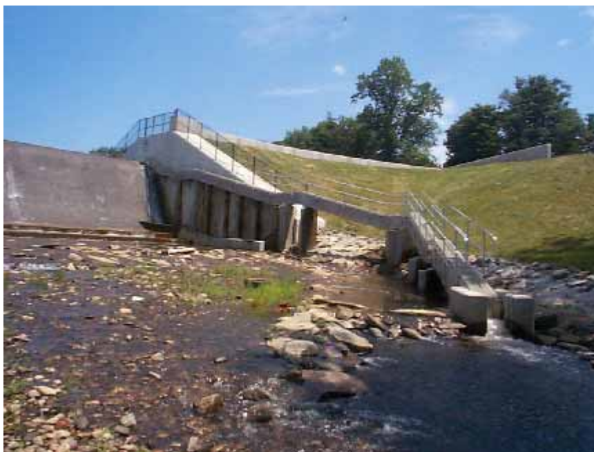
Bunnell's Pond Dam and newly installed fishway.
