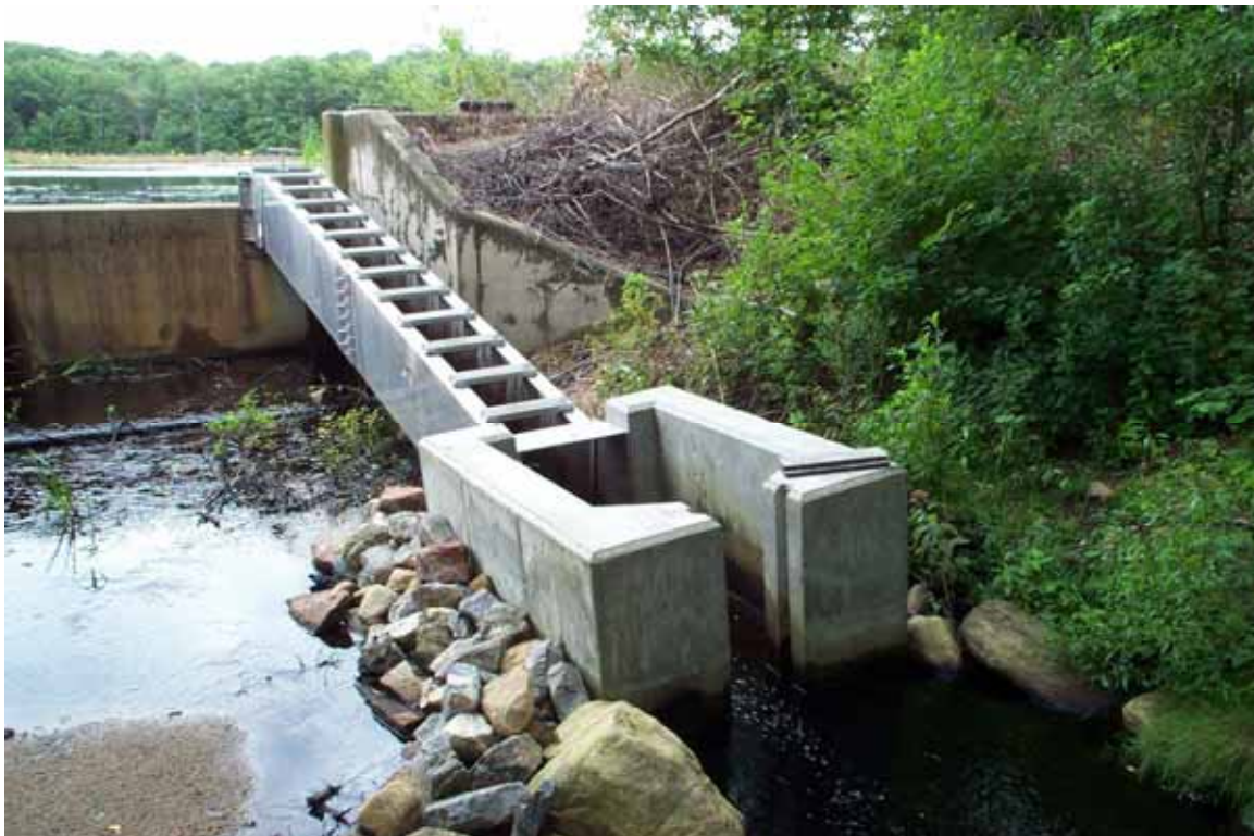
Beaver Swamp Brook Dam and newly installed fishway.
