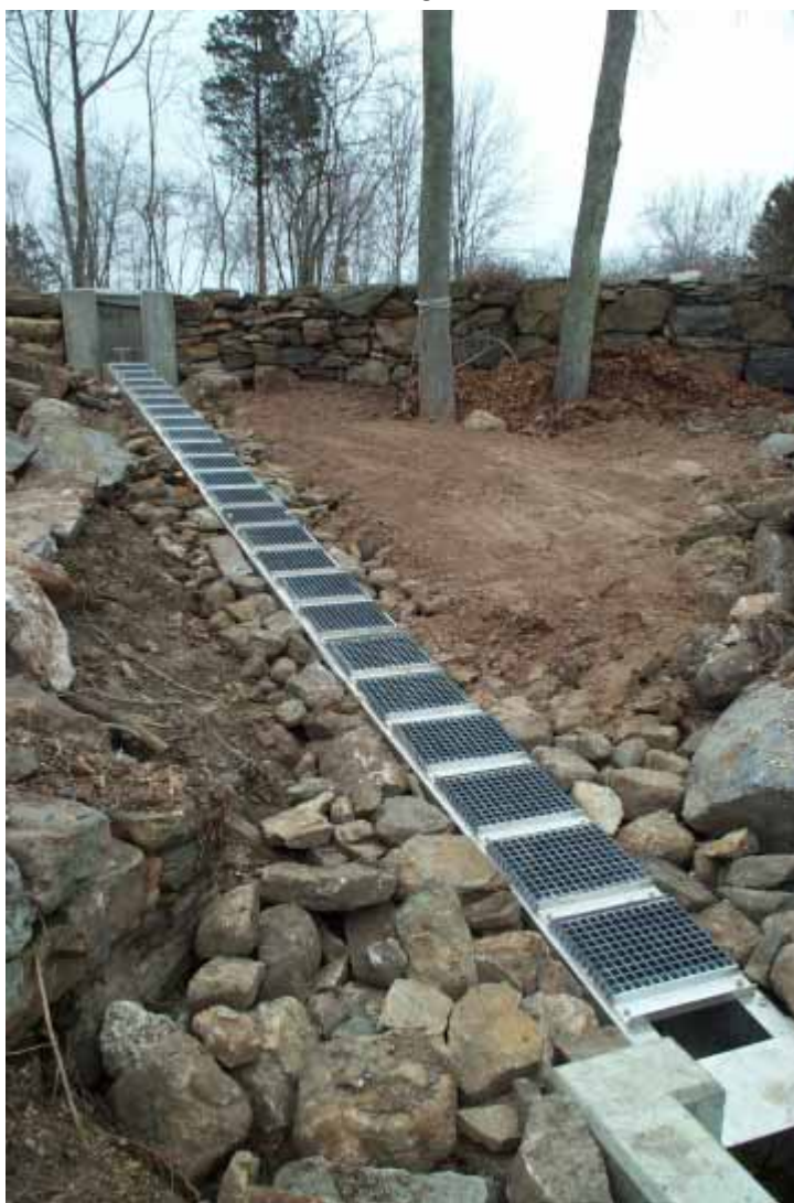
Construction of the fishway on Upper Millpond Dam.
