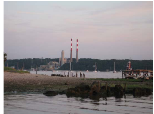
Port Jefferson Harbor, LIPA Plant and STP
