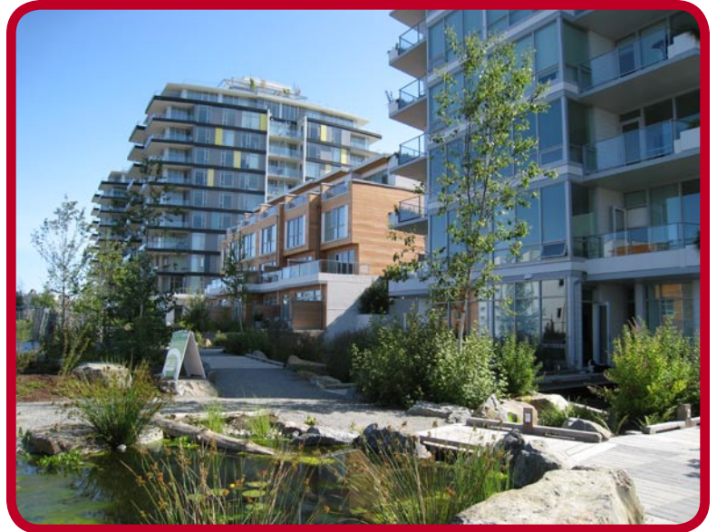
Onsite stormwater management , such as this passive water feature in Victoria, BC, is one example that will be replicated in Bridgeport.
