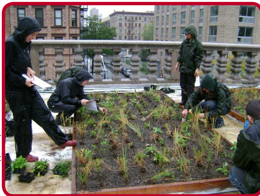
GreenApple Corps members install green roof structures at The Jackie Robinson Recreation Center in Harlem, NY.
