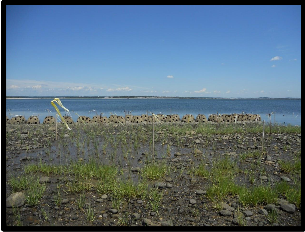
Panoramic view of the reef balls and tidal marsh restoration site. (photo credit: Amy Mandelbaum)
