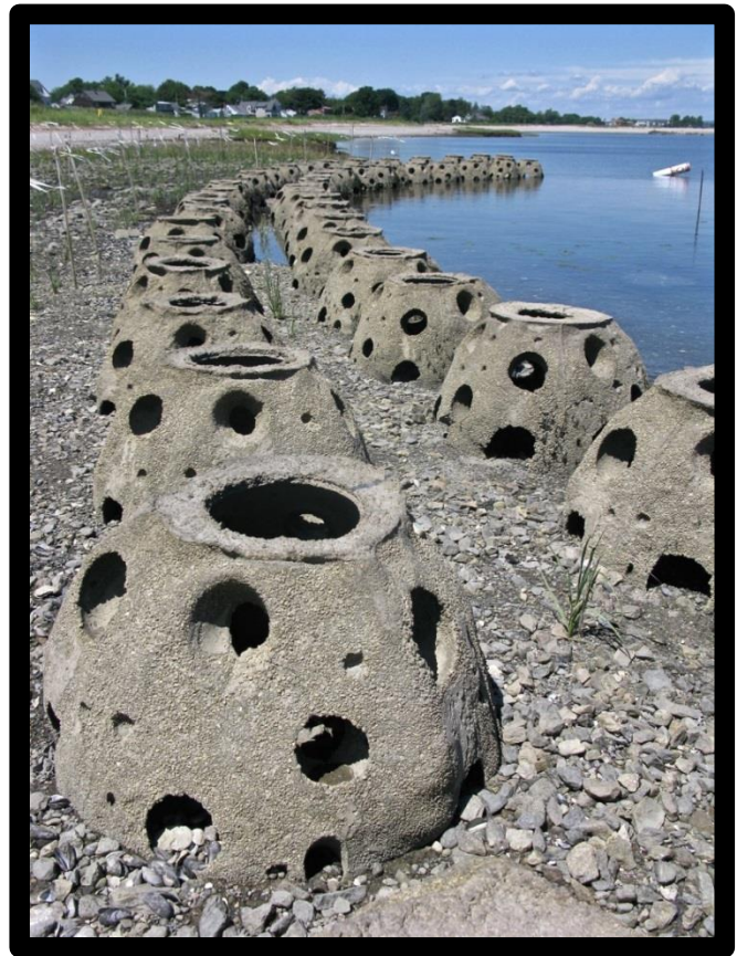
A close up view of the reef ball structures at Stratford Point. Newly installed tidal marsh plantings can be seen landward of the reef complex. (photo credit: Judy Preston)
