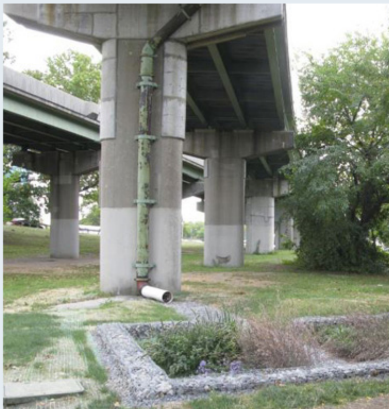
One of two demonstration that divert stormwater from the Van Wyck
