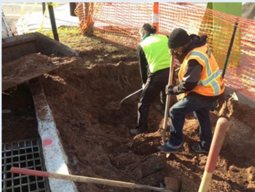
Urban Resource Initiative's GreenSkills crew in December building the first of eight residential bioswales to divert stormwater runoff in New Haven.
