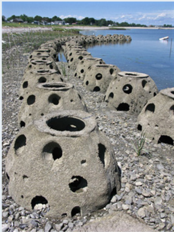
Some of the concrete reef balls being used to stabilize the Stratford Point shoreline.
