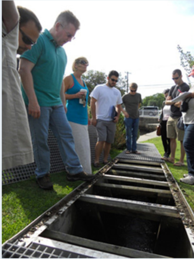
Workshop attendees inspect a newly installed fishway at Argyle Lake in Babylon, NY.
