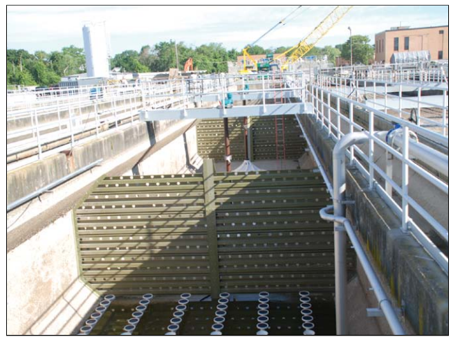
Figure 1. Stratford aeration tank.
