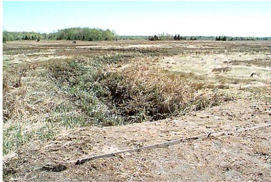
Photo showing a ditch segment that is plugged with soil from a nearby pond. Plug is in the foreground.
