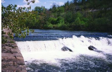
**Cause of Degradation:** Timber Crib Dam which obstructs fish passage.
