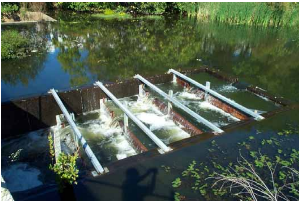
Clark Pond Dam Fishway as seen from above.
