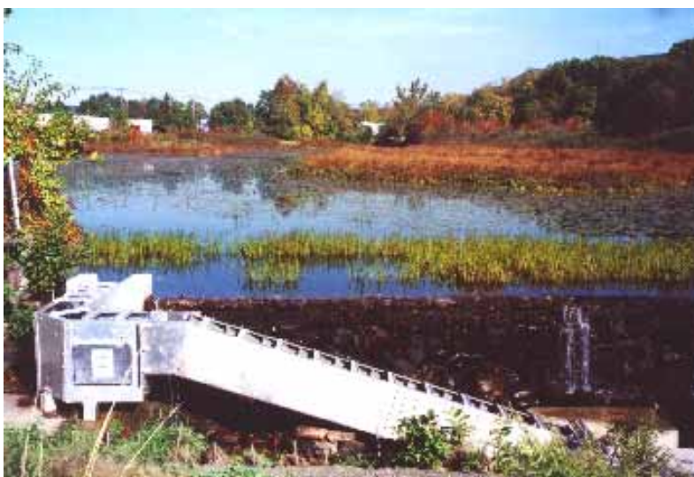
A view of the fishway installed on the Pond Lily Dam, looking upstream (north) into Lily Pond.
