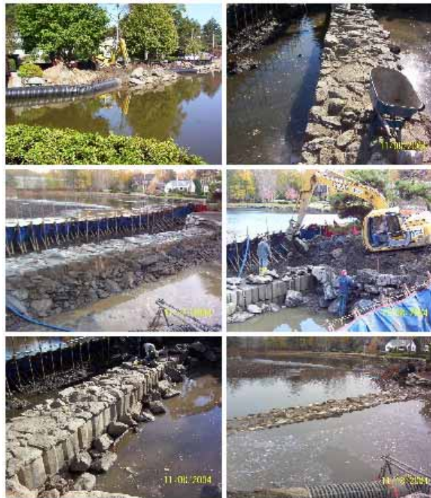
Various stages of construction at Gardens Lake – source:
