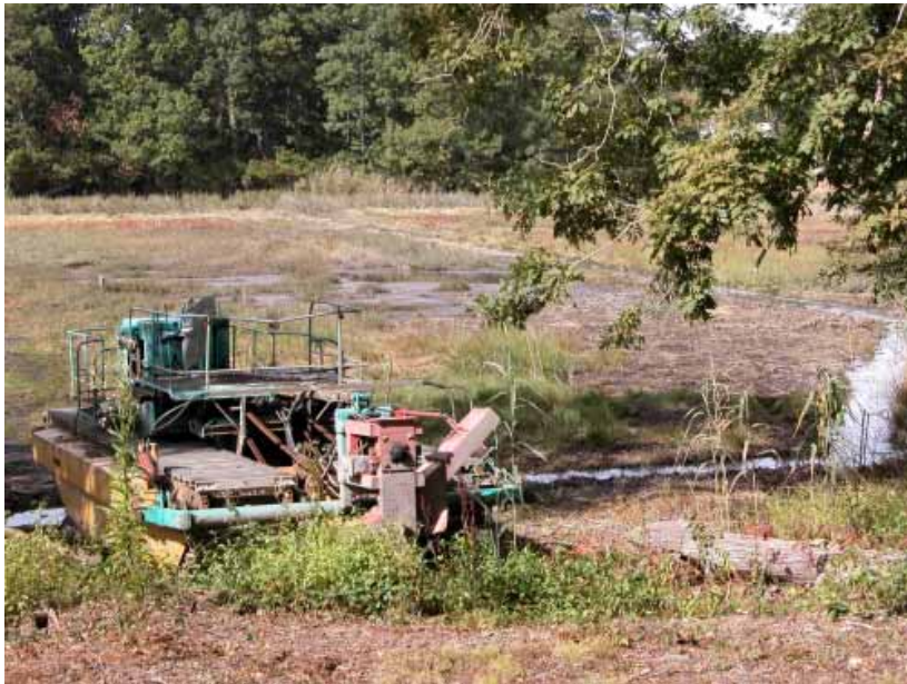
Above: Aerial view of the mouth of Mile Creek. Left: A low-ground-pressure mechanical excavator rests beside one of the tidal wetland panels.
