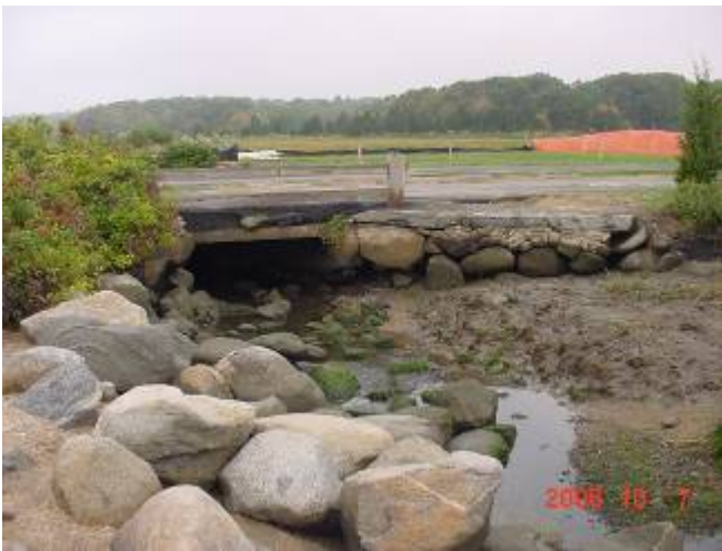
Top image shows the pre-existing culvert and the bottom photo shows the new culvert that better allows adequate flow. Photos Courtesy of CT DEP.
