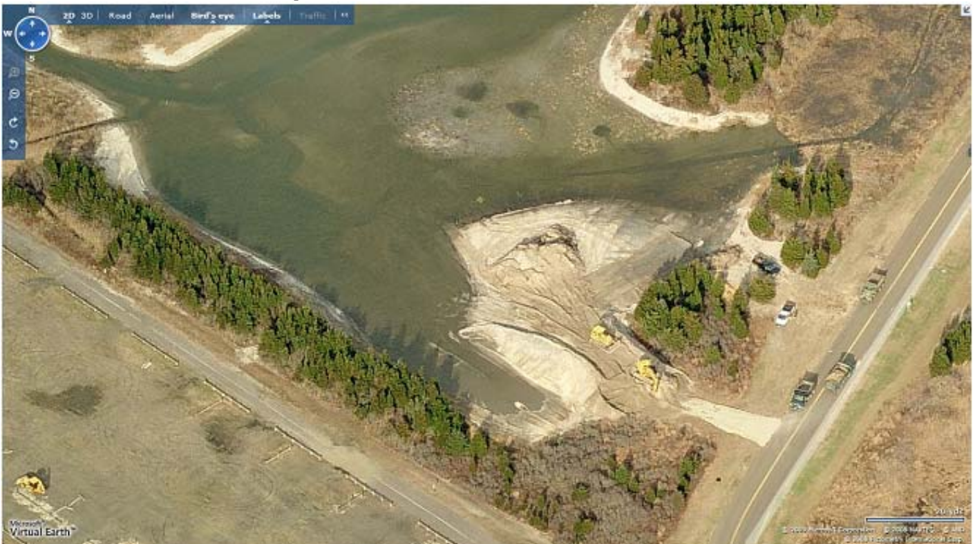
Hammonasset Beach State Park wetland restoration project under construction.
