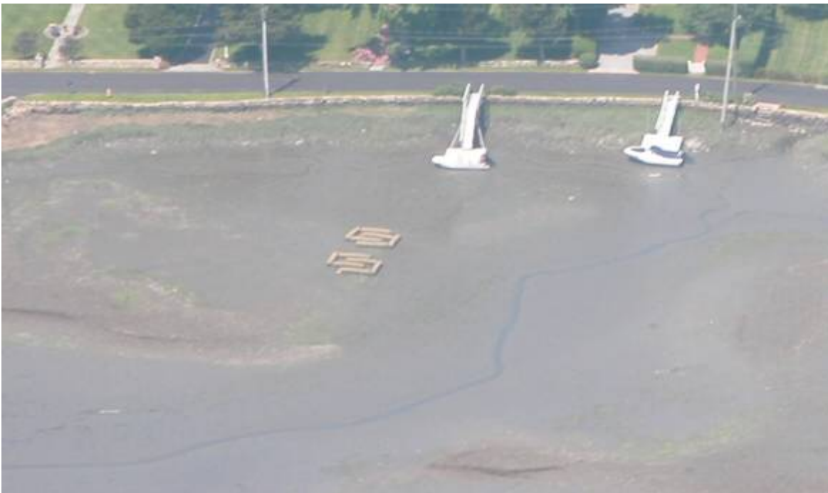
This aerial photo shows the maze-like arrangement of coir logs in the Fivemile River which were installed to “baffle” tidal waters, slowing the velocity and promoting sedimentation.
