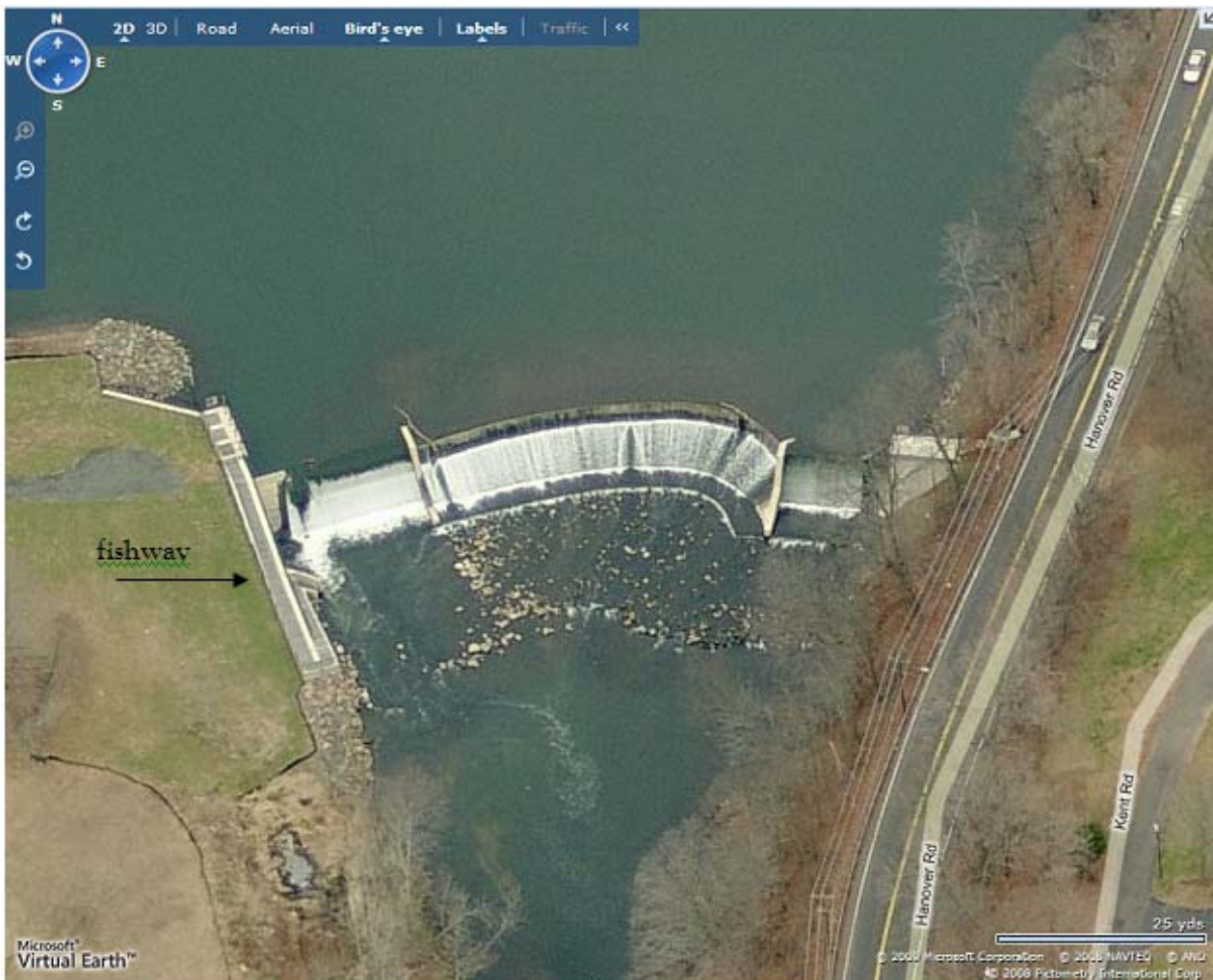
Hanover Pond Dam with fishway installed along the west side.
