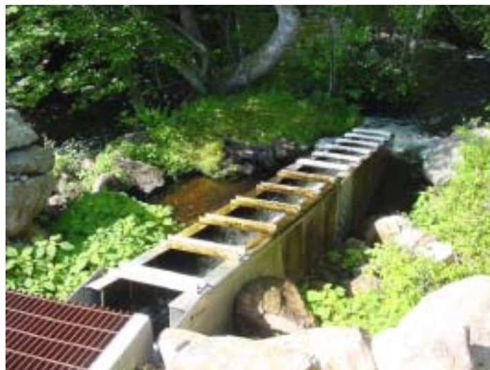
Steepass fishway unit added at Hyde Pond Dam
