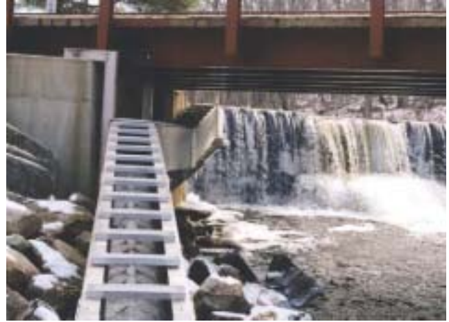
Steppass fishway installed beneath a town bridge
