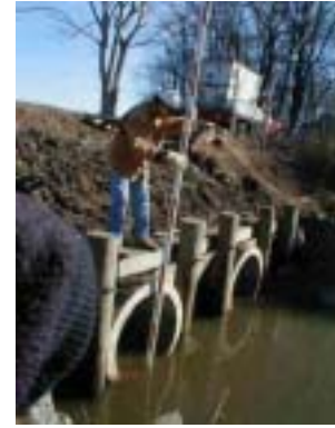
Checking elevations of newly installed pipes
