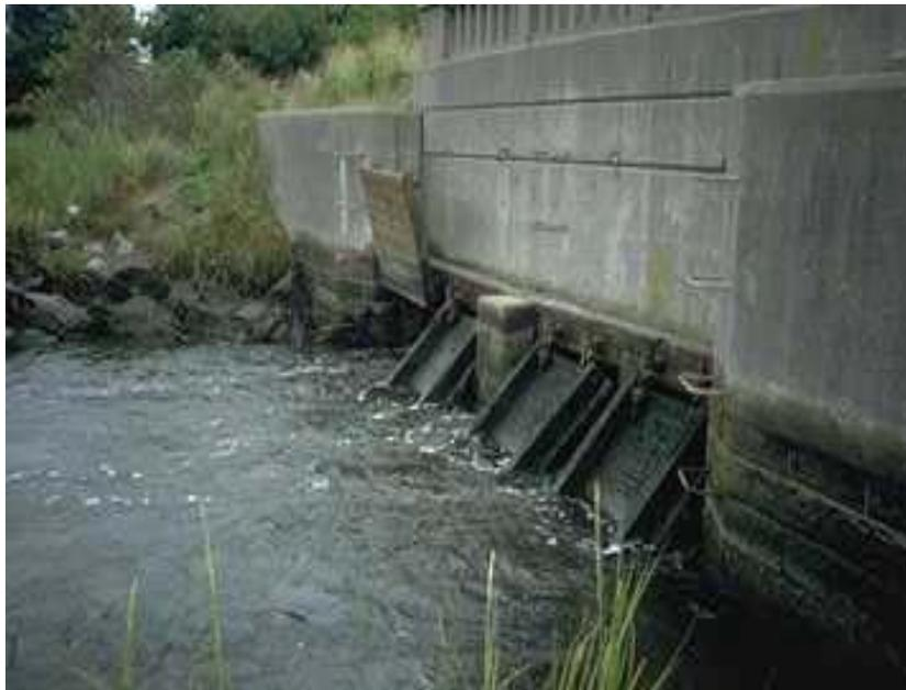
One of four flap tide gates was opened at Hammock River in Clinton, Connecticut. If more than one gate was opened, it could cause flooding of low-lying residential properties built close to the wetland.
