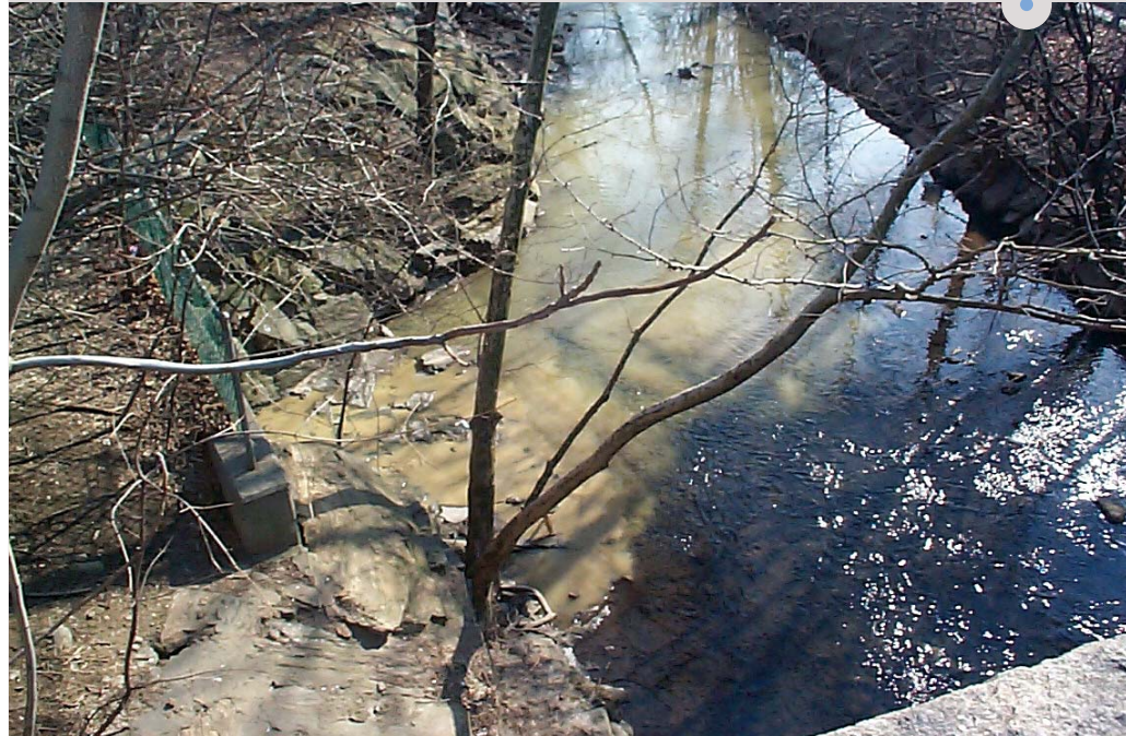
An outfall pipe, below fence, discharges sediment into the Bronx River.
