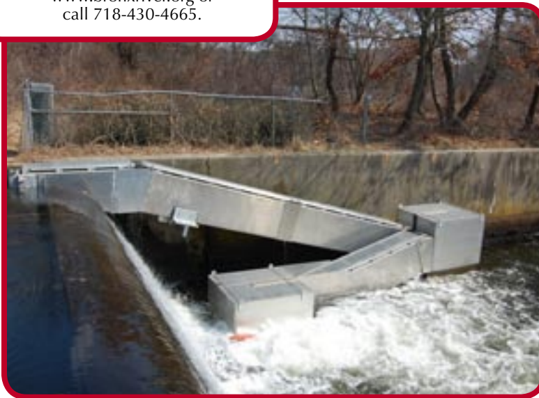
This fish ladder allows migratory fish access to habitat upstream of a dam on the Carmans River, Long Island, NY.
