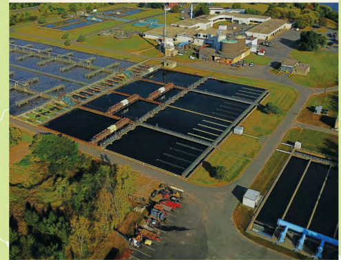
Enhancing Nitrogen Removal at the Springfield Regional Wastewater Treatment Facility (MA)
