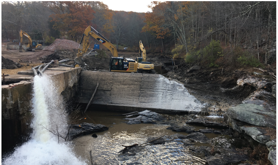
A dam no longer in use and former paper mill were removed. The restored stream bed has now opened up 17 miles of fish migratory habitat.
