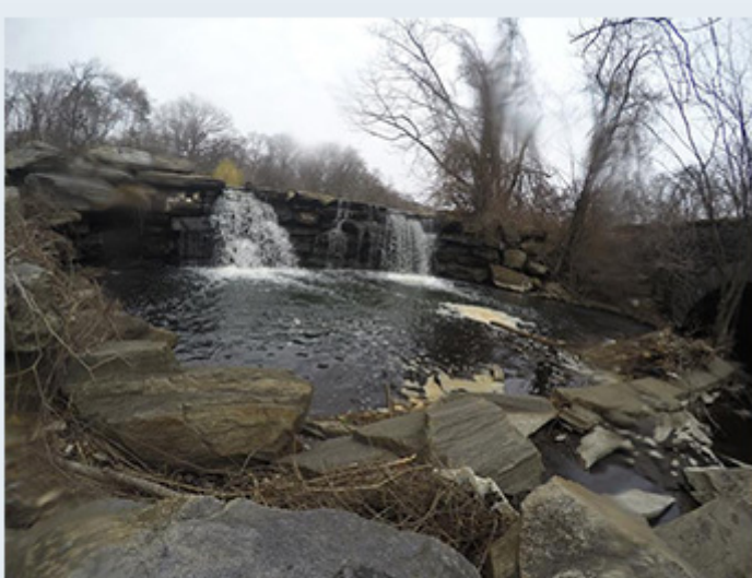
The Pelham Lake Dam in Mount Vernon, NY.
